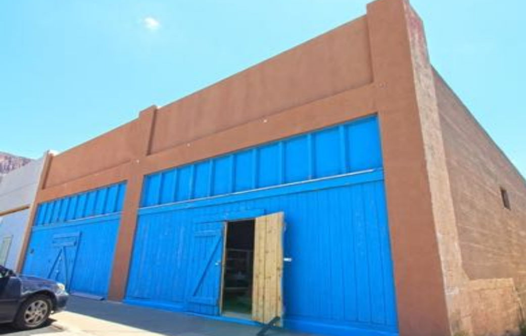
Exterior of Building
