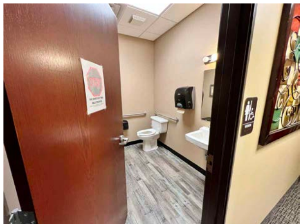
603 A - 1 of 2 Restrooms
