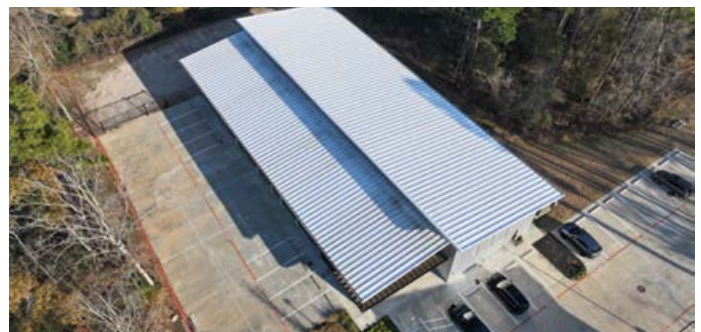
Standing seam metal roof and efficient site configuration.
