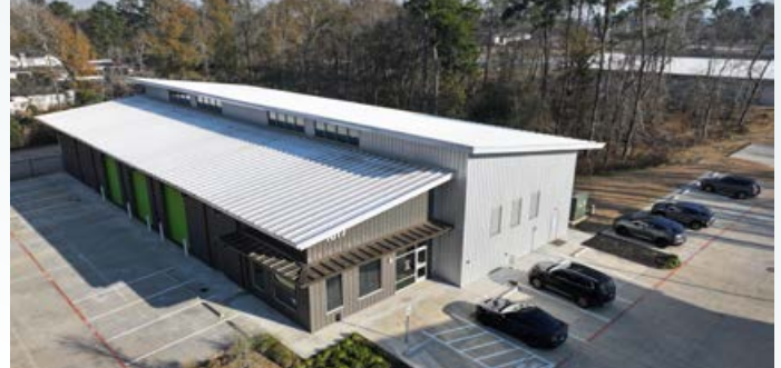
Storefront entry and dedicated parking.
