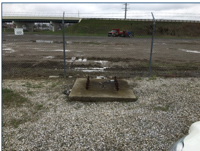
Pedestal with conduit for pylon sign
