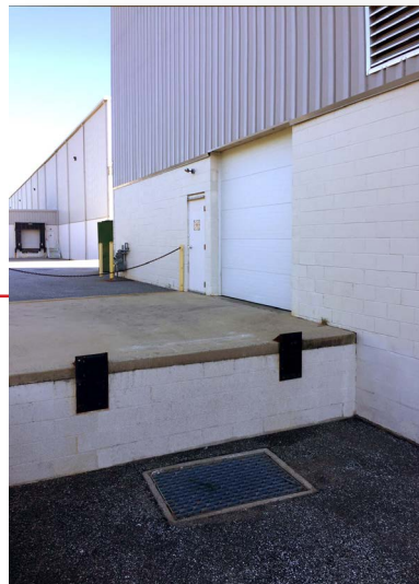
Dock with Concrete Pad and Overhead Door
