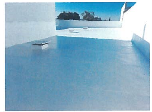
New Silicon Roof Coating
