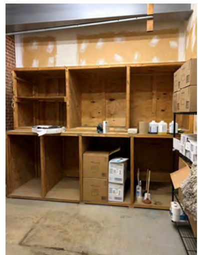
Garage Storage Area
