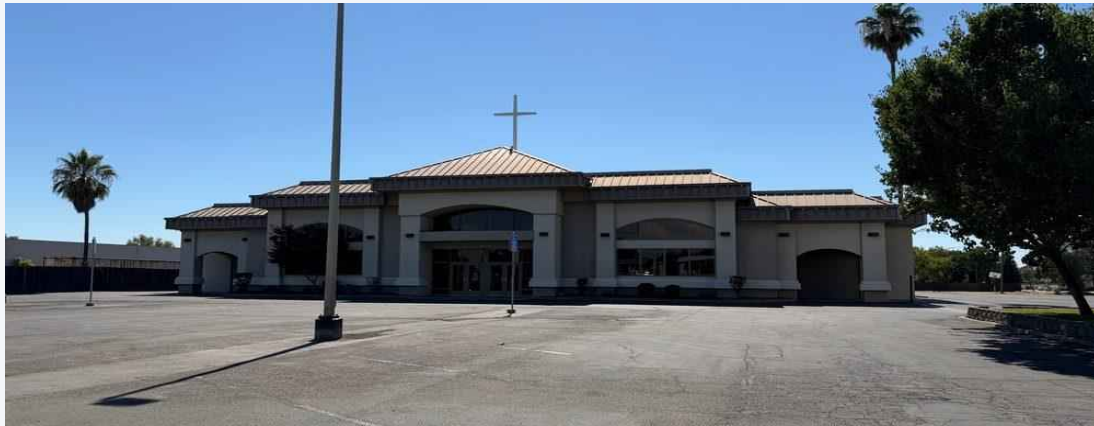
Primary elevation & monument frontage on Watt Avenue
