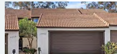
2062 AVENUE OF THE TREES NEAREST TO PROJECT SITE
