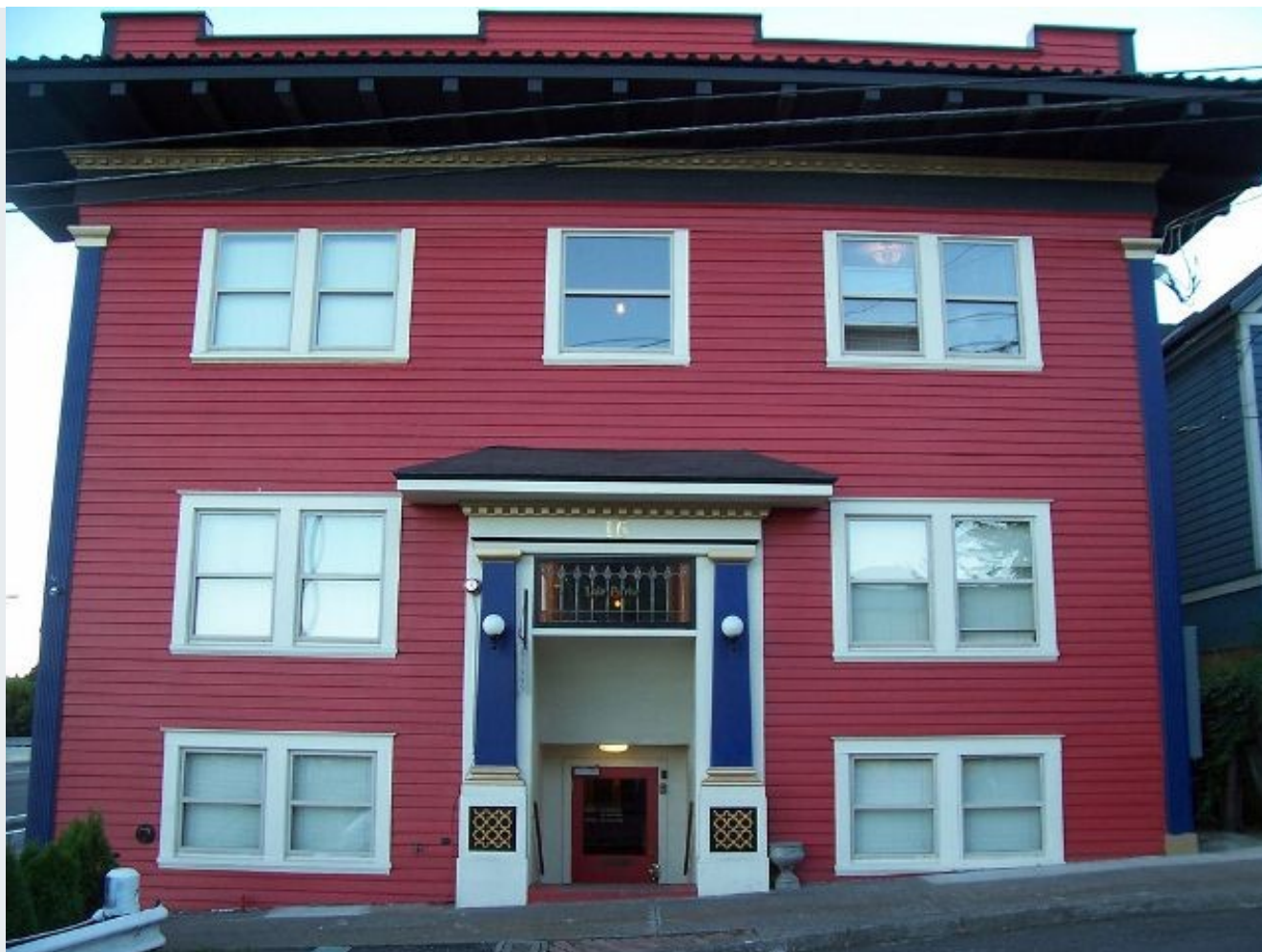
Front exterior view
