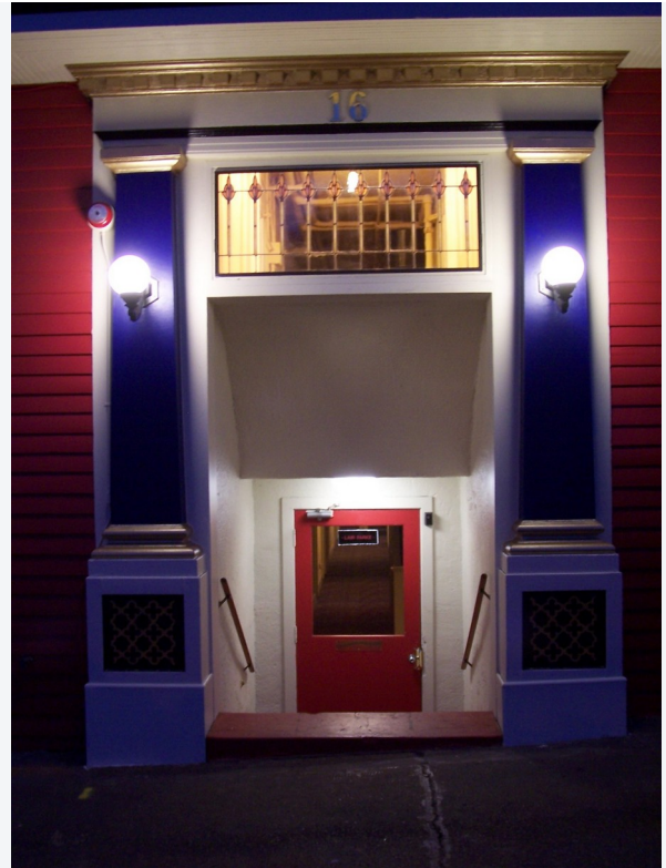
Main entry architectural detail
