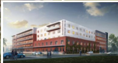
WAREHOUSE DISTRICT RE-DEVELOPMENT 800 BLOCK, WILLIAMS @ McKEE ST
