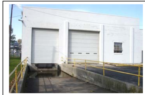
East Receiving Area
