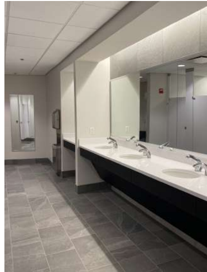
LOBBY MODERNIZATION Common Corridor & Restroom Upgrades
