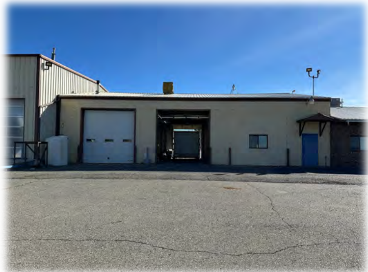
North Shop Overhead Doors – 12' x 12' (Size common to all overhead doors)
