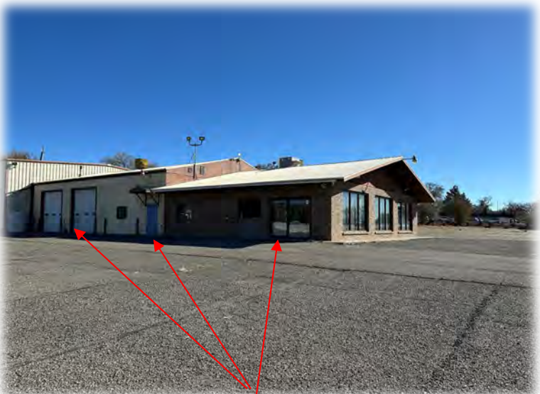
Office North Exterior Door and Overhead Shop Doors
