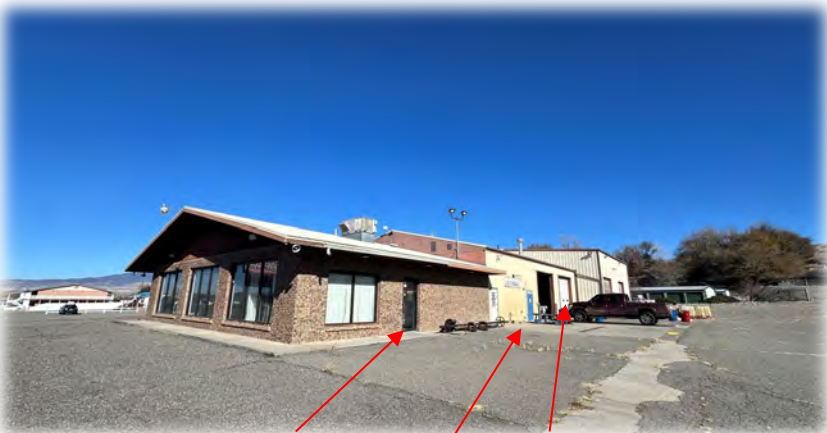
Office South Exterior Door and Shop Exterior and Overhead Doors
