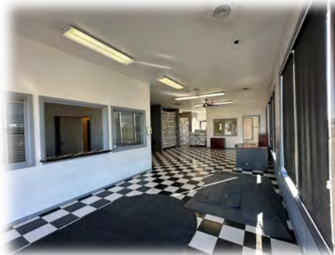
Lobby Looking South
