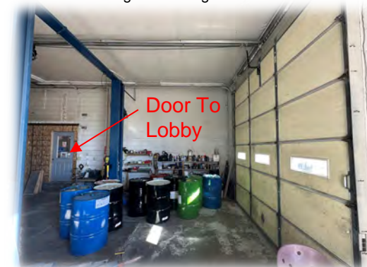
Shop showing Lobby entrance door
