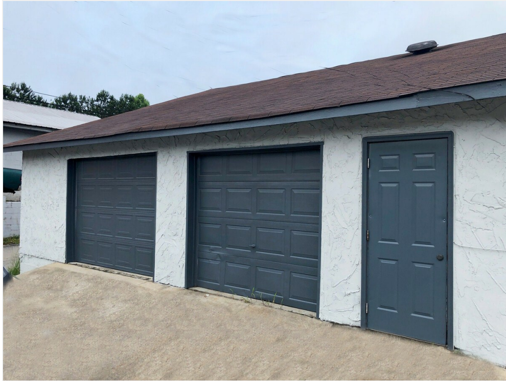
Rear garage of front building
