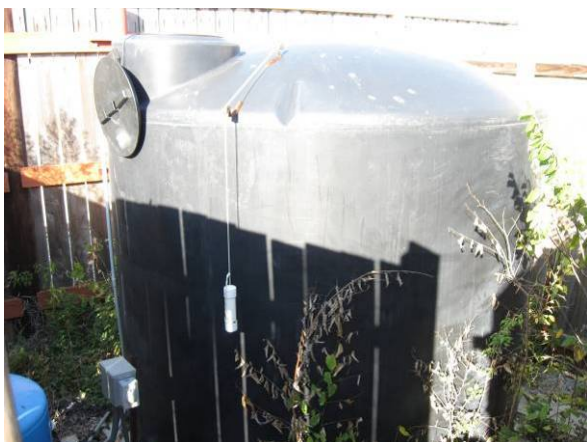
Photo #5 Photo showing the water storage tank on the site. Note the blue pressure tank left of the water tank.
