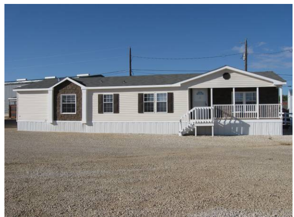
Photo #6 Photo showing typical demonstration home on the site.
