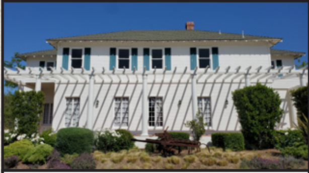
Building D - Existing 2,000 SF Historic Johnson-Ward House
