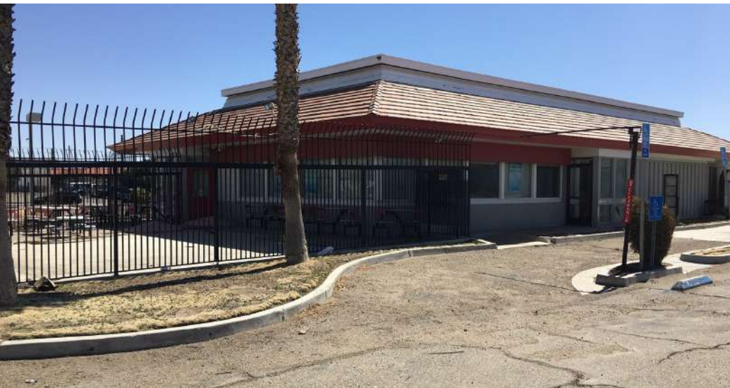
Pad Building - Former Carl's Jr
