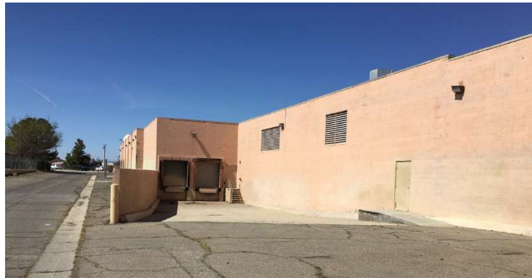
Back of 21671 - Loading Dock
