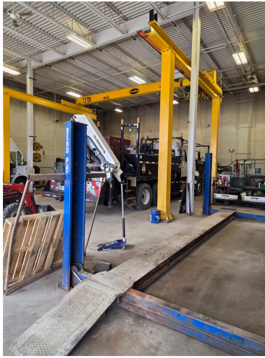
Rear shop — crane overhead
