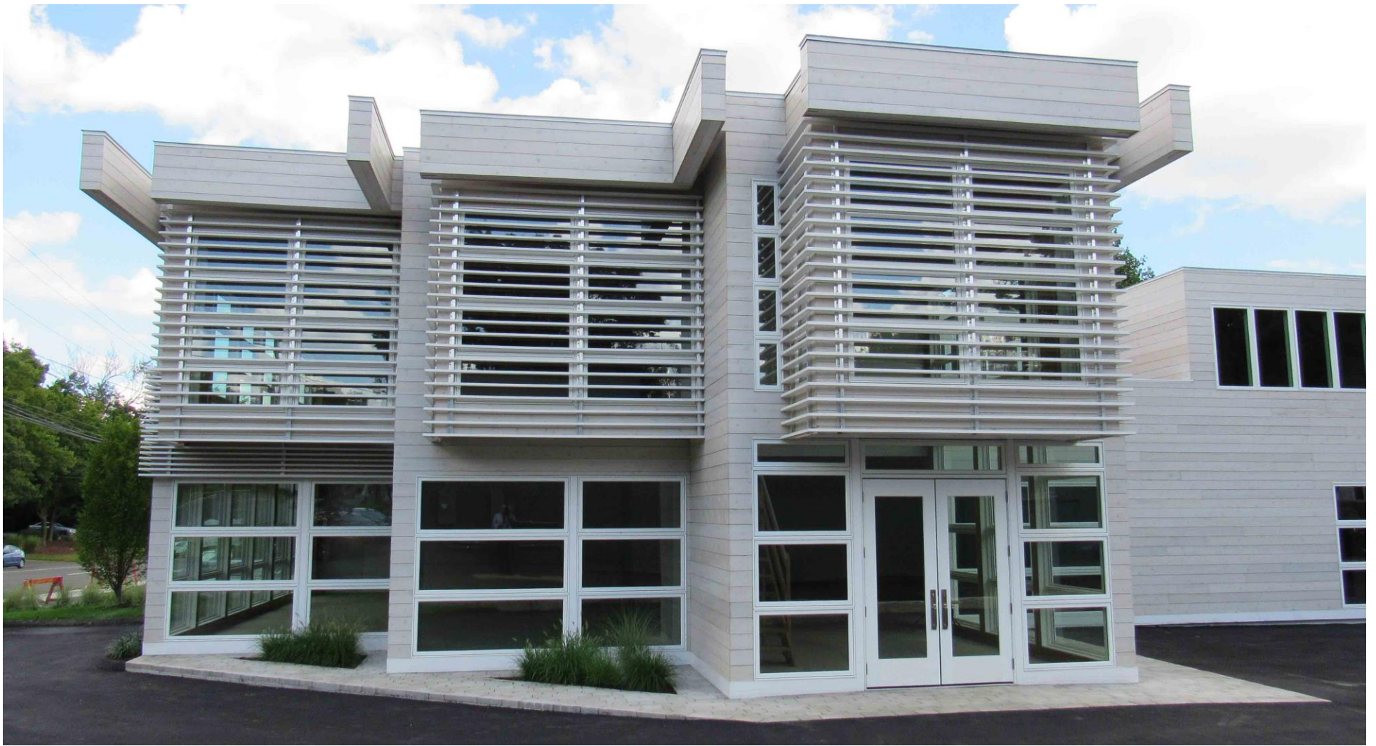
Side building view and main entrance
