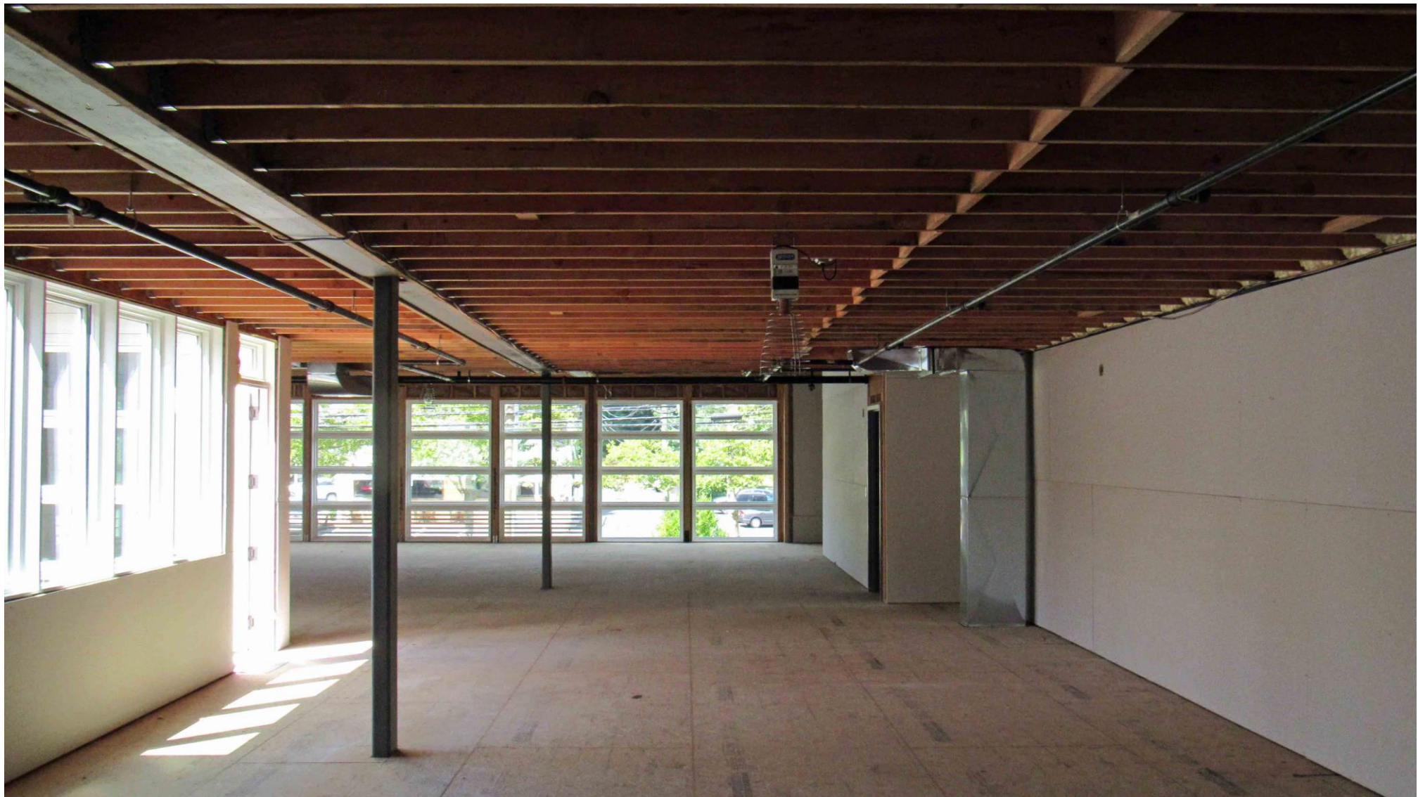
Second floor interior
