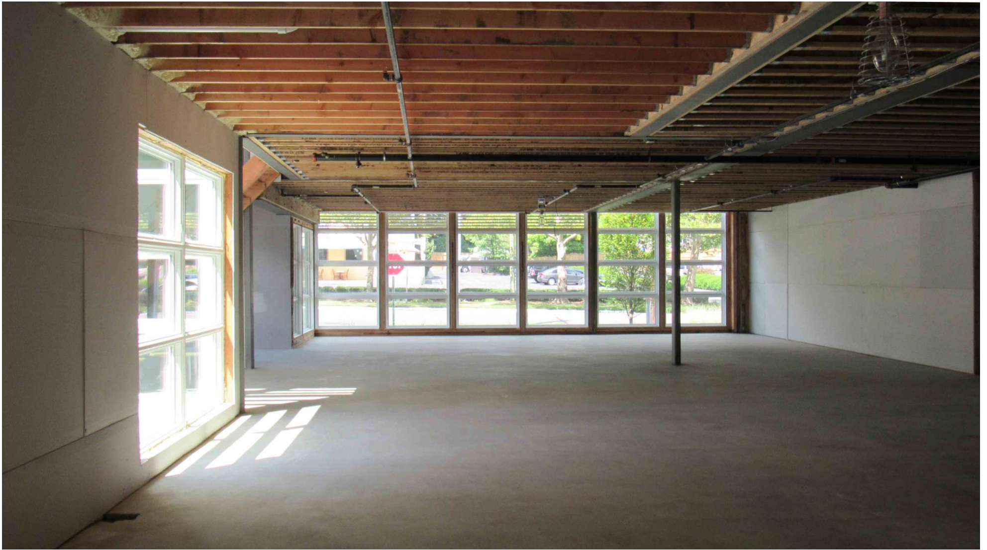
First floor interior
