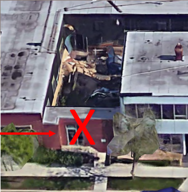
Existing Link / Courtyard
