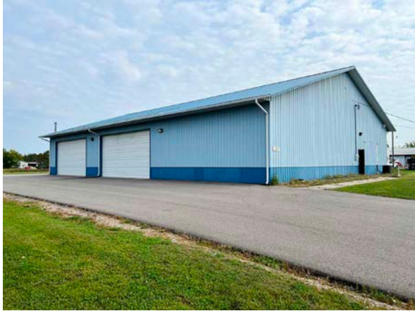
SW Corner of Building
