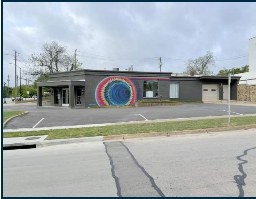
NORTH SIDE OF SUBJECT BUILDING
