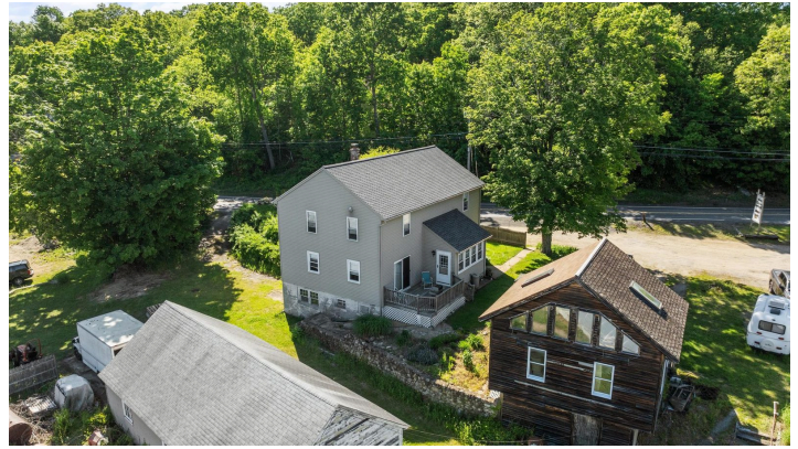
Residence, detached garage and accessory building on Lot 3
