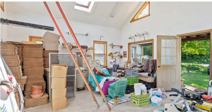
Accessory building — vaulted ceiling, skylights & windows
