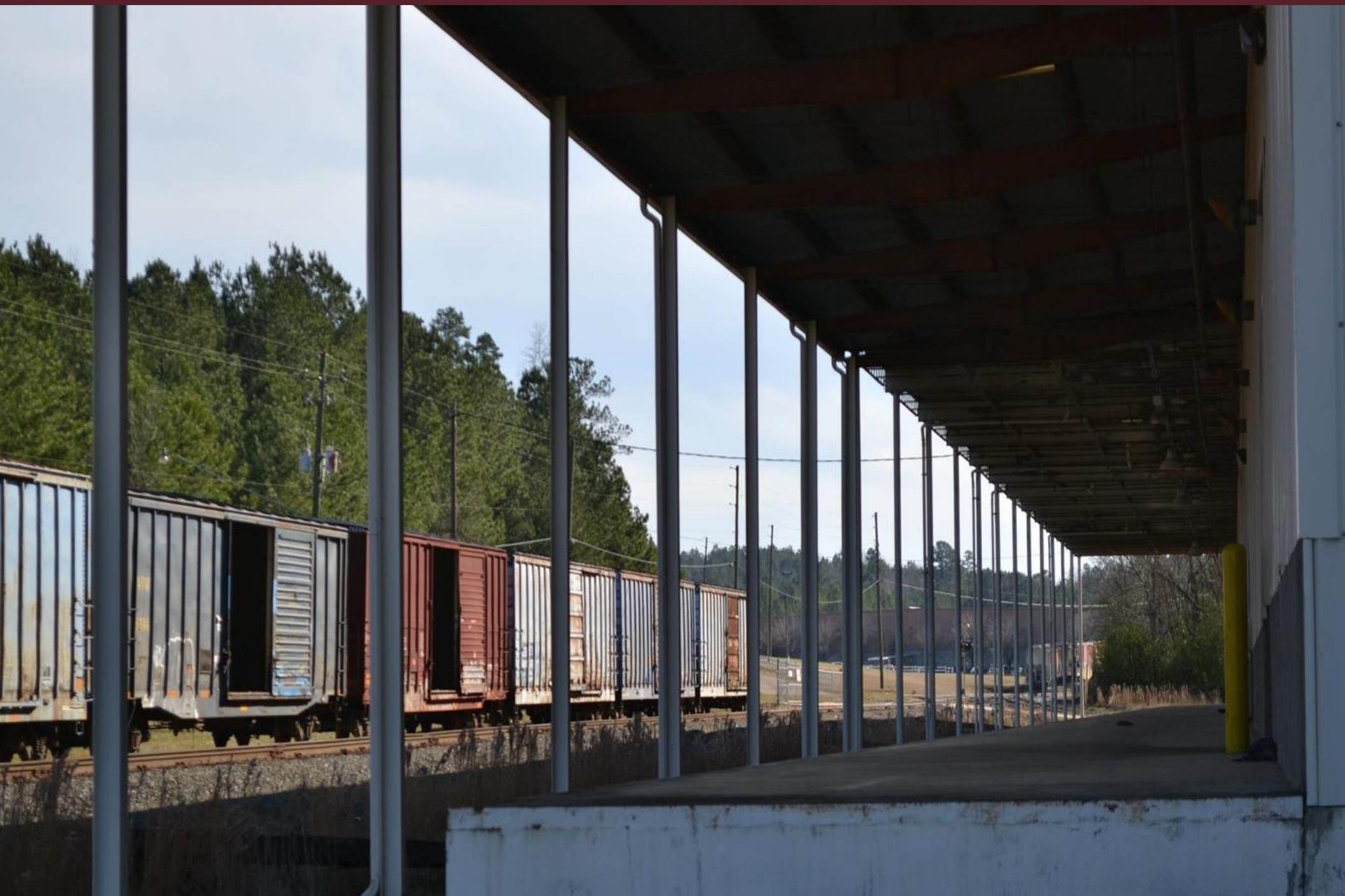
Rail Line 9 Cars
