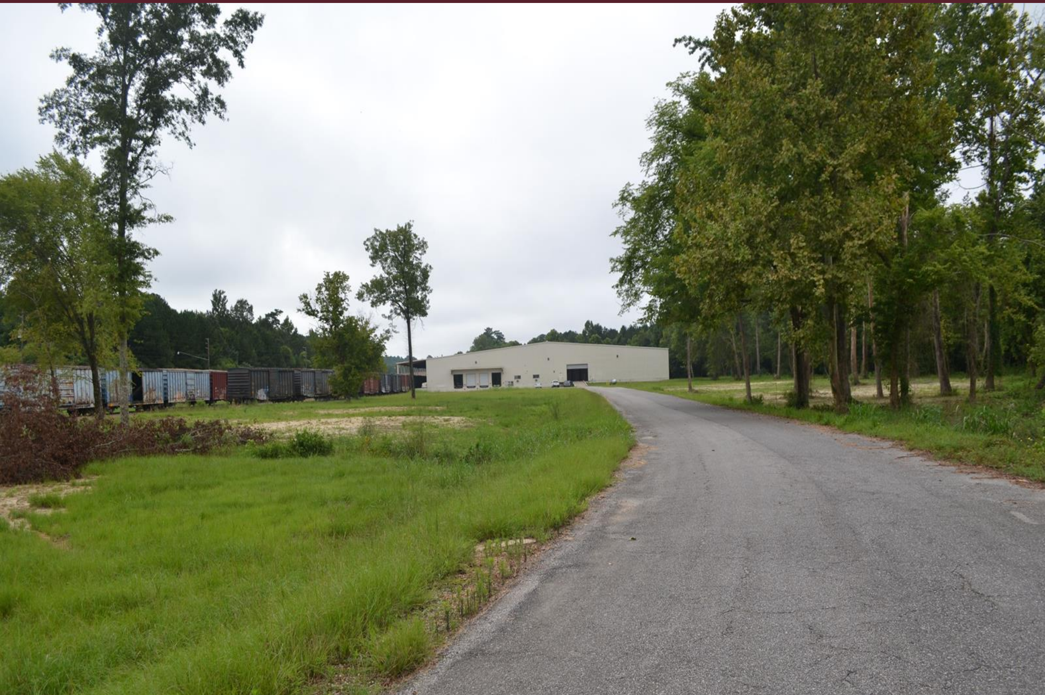
Private Entrance Road
