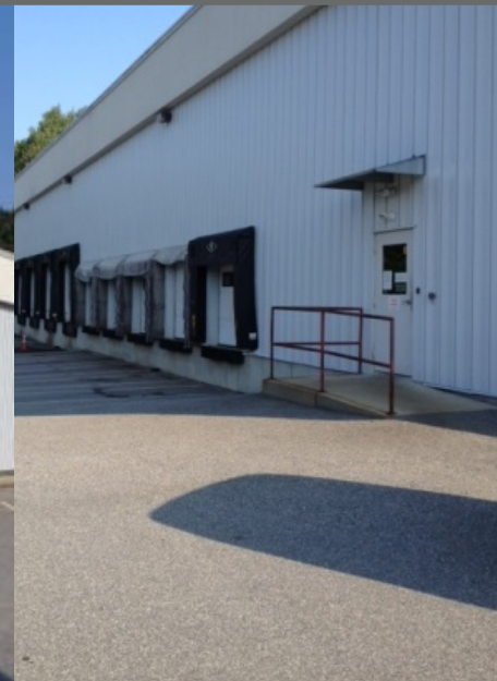
HIGH BAY DISTRIBUTION FACILITY
