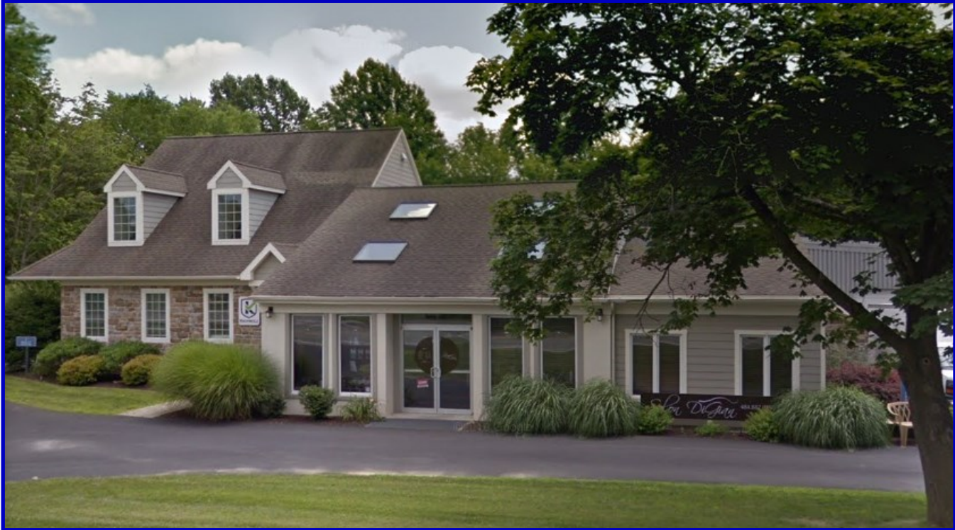
VIEW OF WHOLE BUILDING
