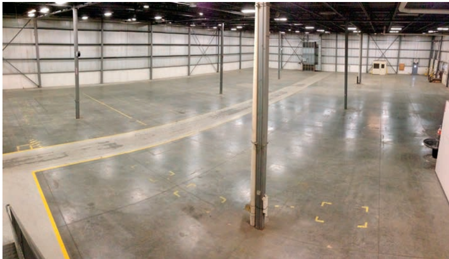
New Addition - Warehouse
