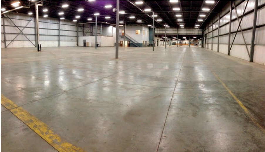
New Addition - Warehouse
