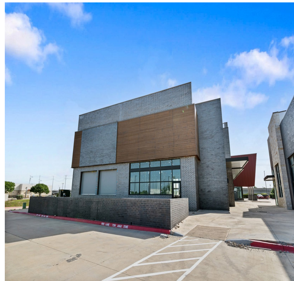
Exterior — Building 1 corner entrance & patio wing
