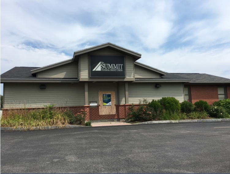
View from NYS Route 31
