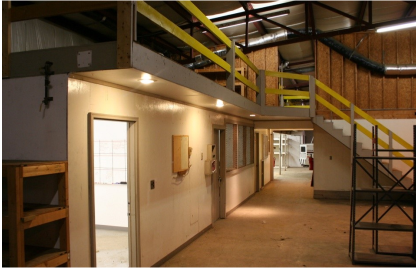
Back Workshops Corridor (From East Bay)
