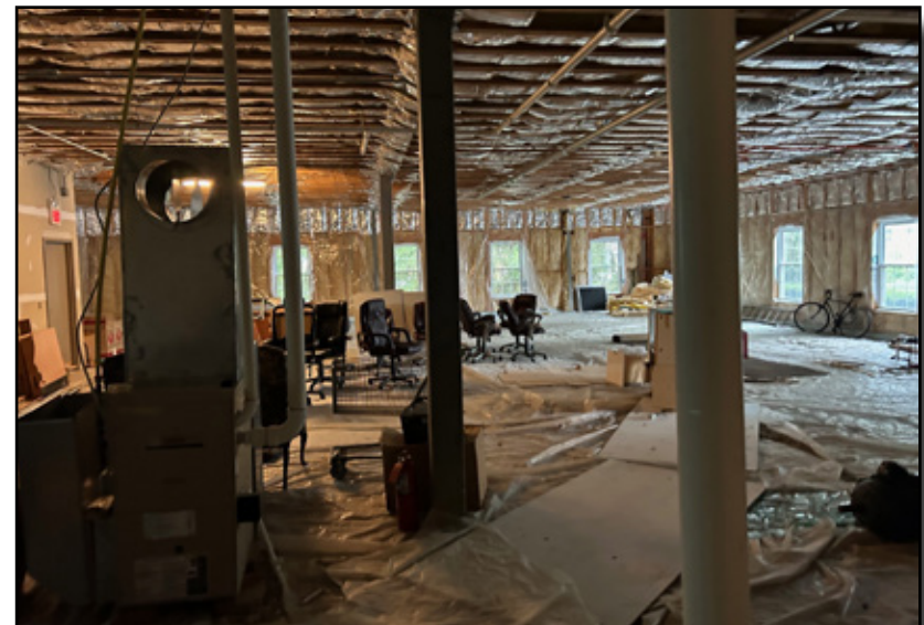
Unfinished Office Space
