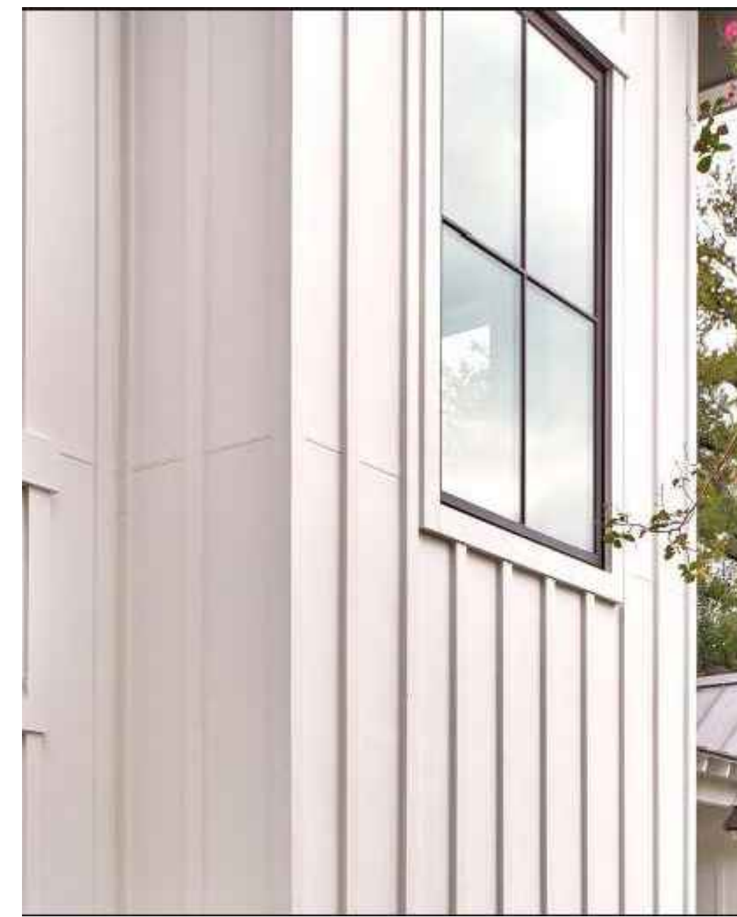
SIDING - BOARD AND BATTEN, 16" SPACING
