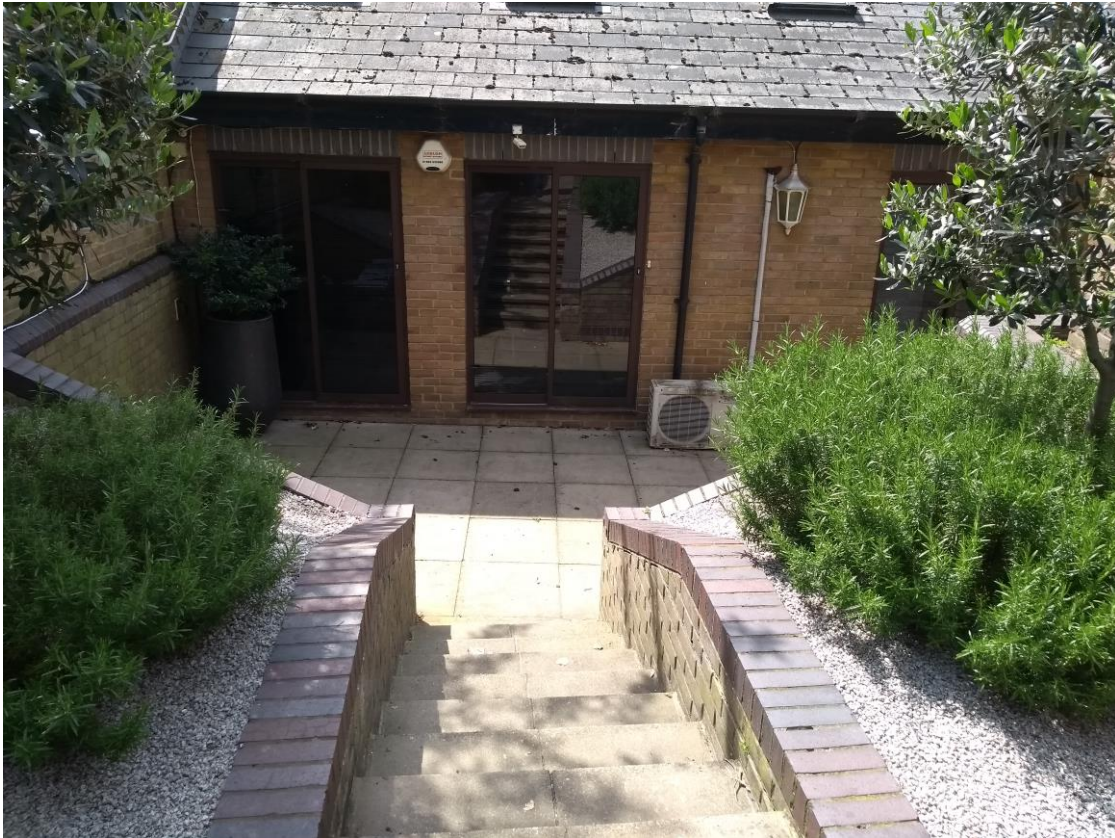
Rear access leading from the car park
