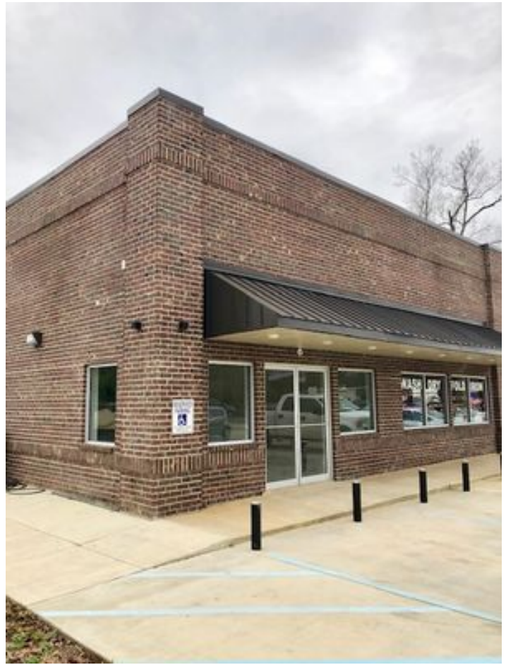
Wired Alarm/Security Systems
