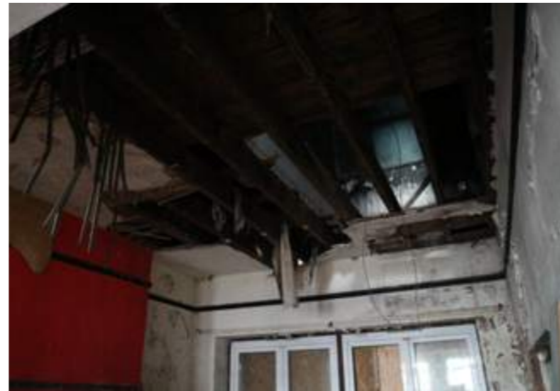
Img. 03 - Ad hoc / later additions like glazed door
