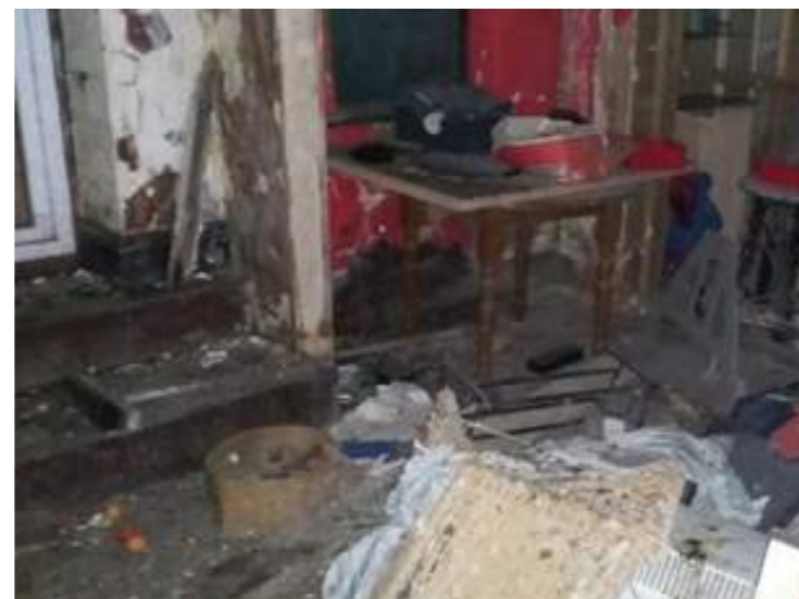
Img. 06 - Existing internal ad hoc construction
