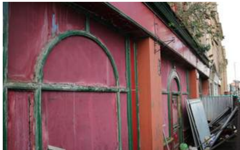
Img. 03 - Existing shopfront behind hoarding
