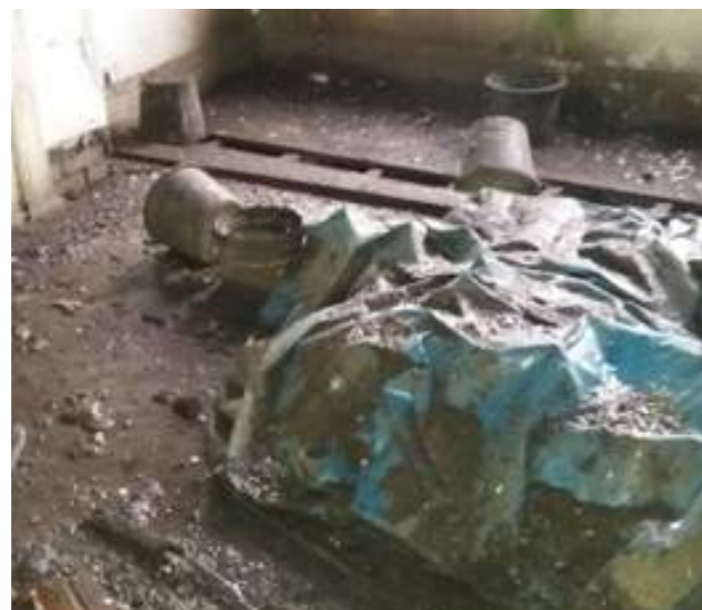
Img. 05 - Typical internal condition
