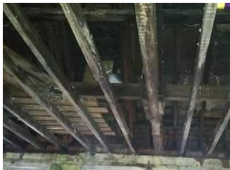
Img. 07 - Internal Ceiling condition
