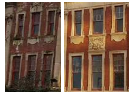
Existing facade condition (L), proposed works to match neighbouring works (R)
