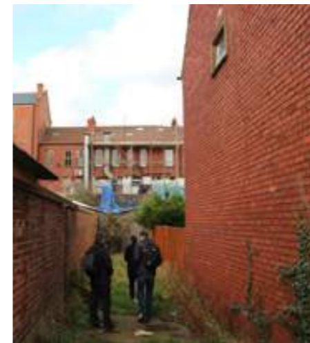
Img. 05 - Rear Access
