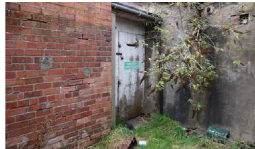
Img. 07 - Rear facade
