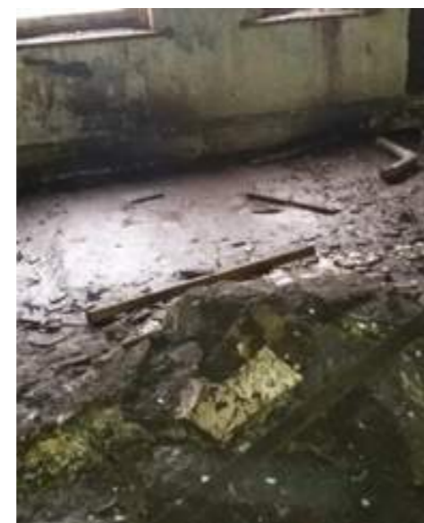
Img. 08 - Typical internal condition
