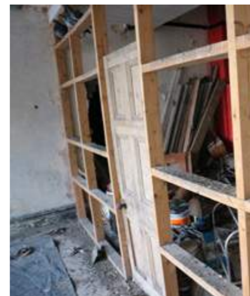
Img. 09 - Ad hoc wall construction
