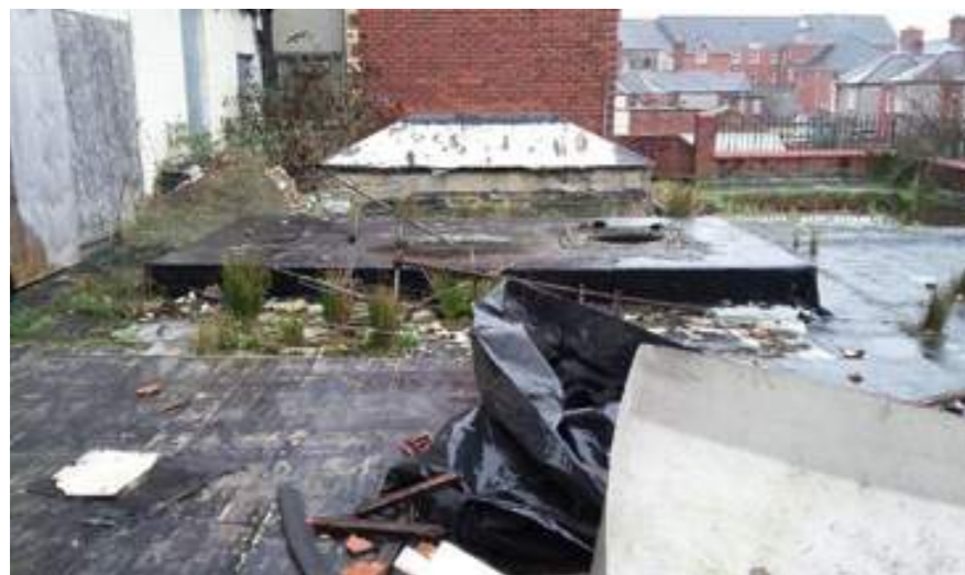
Img. 06 - Existing rear extension roof
