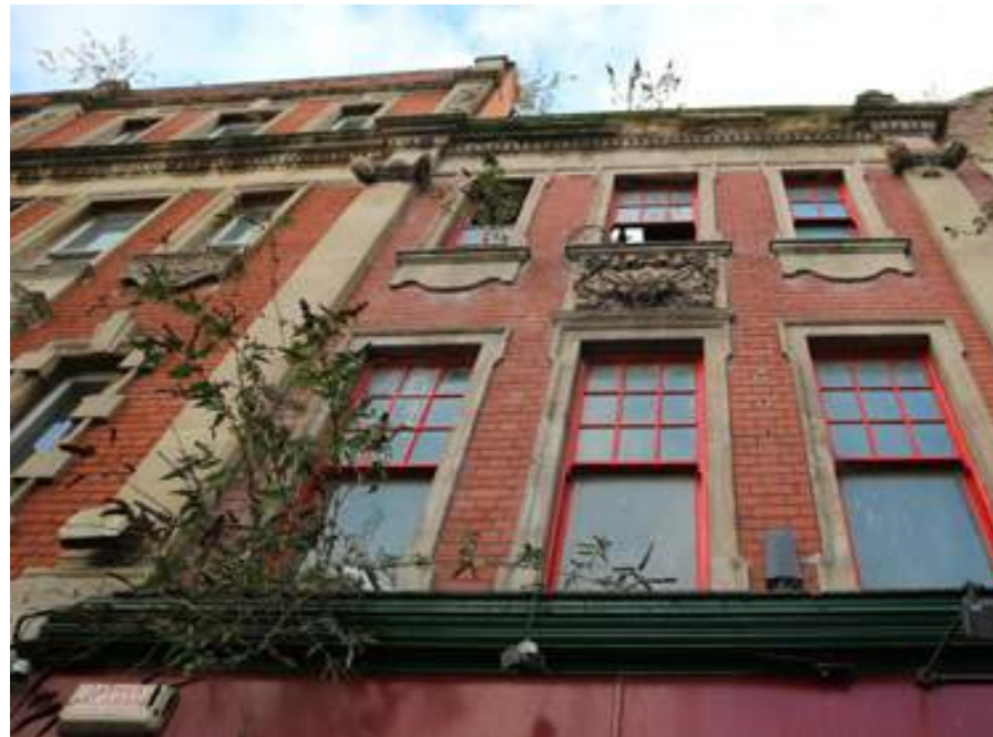
Img. 01 - Front facade detail
