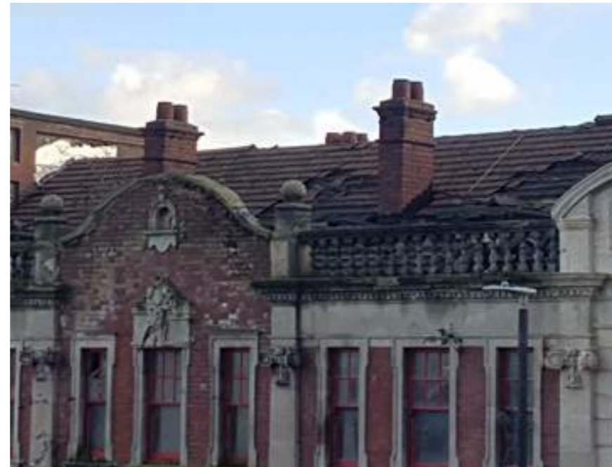
Img. 02 - Roof condition
