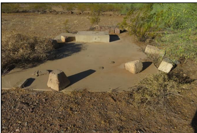
Picture 5 - One of the smaller concrete slabs in the former developed area on the southeast portion of the Property. Remnants of concrete rubble (center) and cinder blocks (top-center) are visible.
