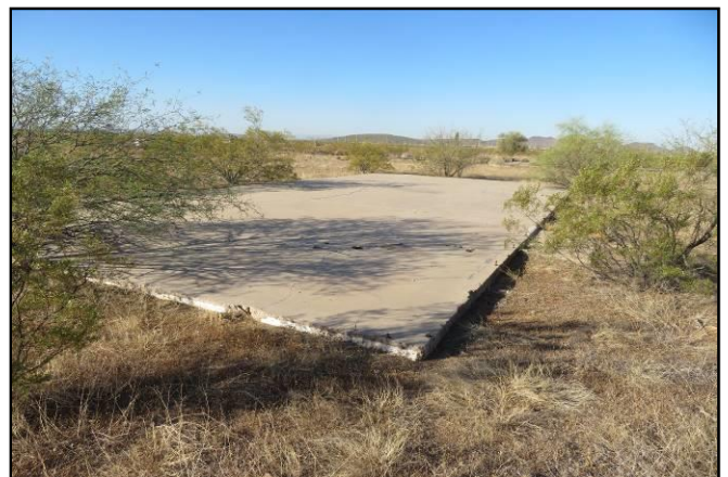
Picture 4 - One of the two larger concrete slabs in the former developed area on the southeast portion of the Property.
