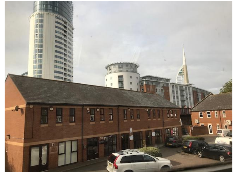
View from first floor
