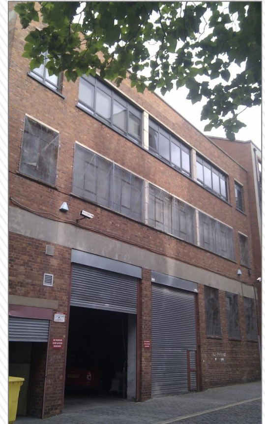
Henry Street elevation including loading bay entrance
