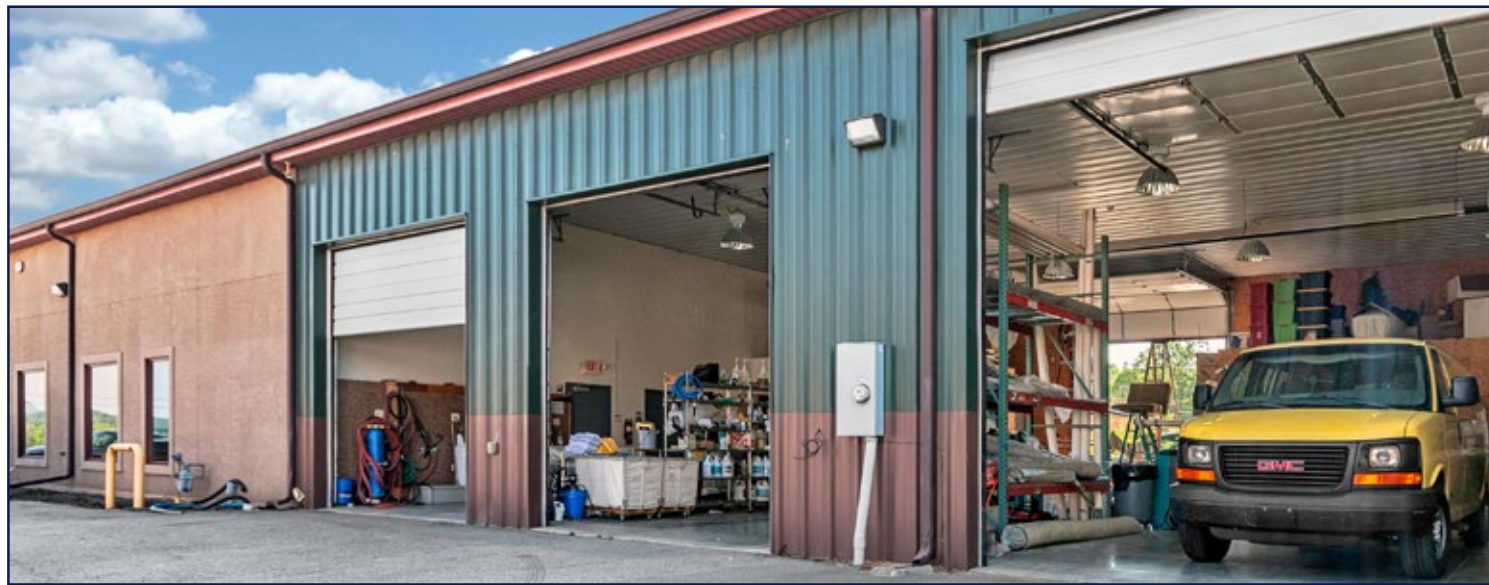
Warehouse section - three of the seven drive-in doors
