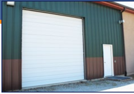
Close up of seventh drive-in door
