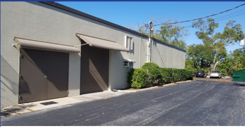
Unit G, East Side of Building
