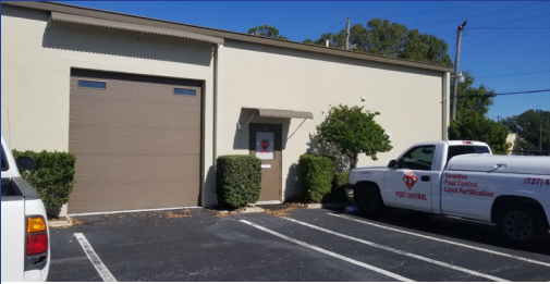
Units F & G, South Side of Building
