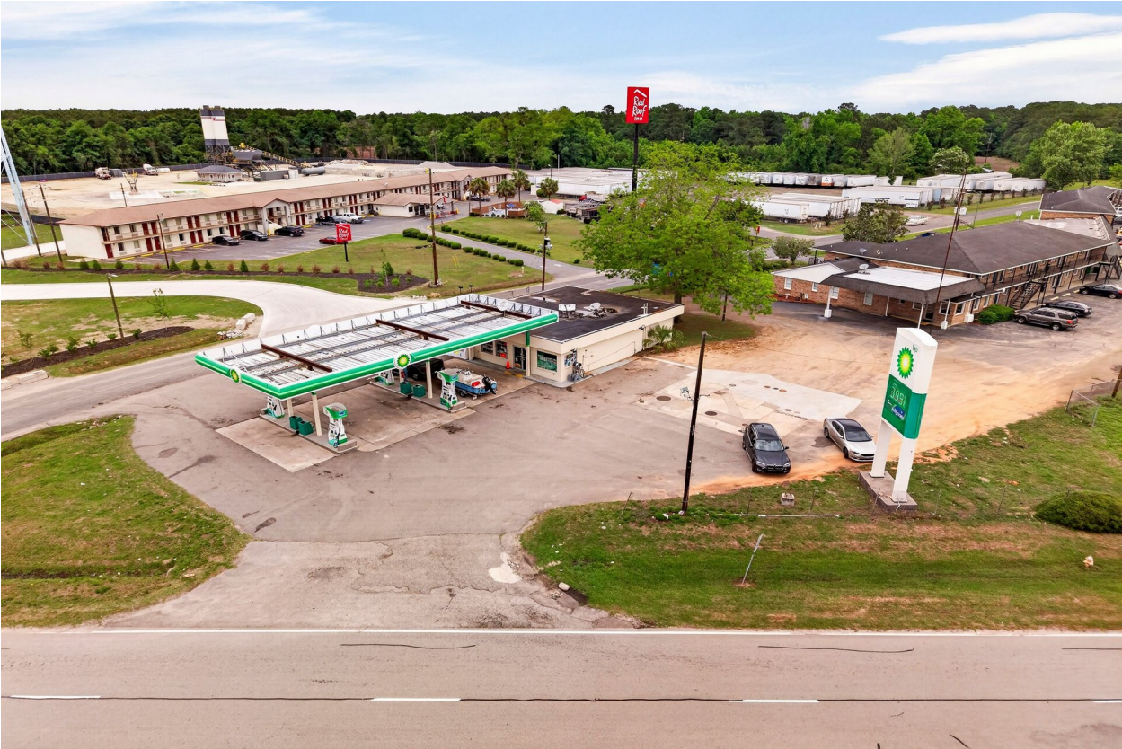
Elevated Aerial — BP Station, Fuel Canopies & C-Store Building | Red Roof Inn Adjacent | Active Fuel Customers Visible
