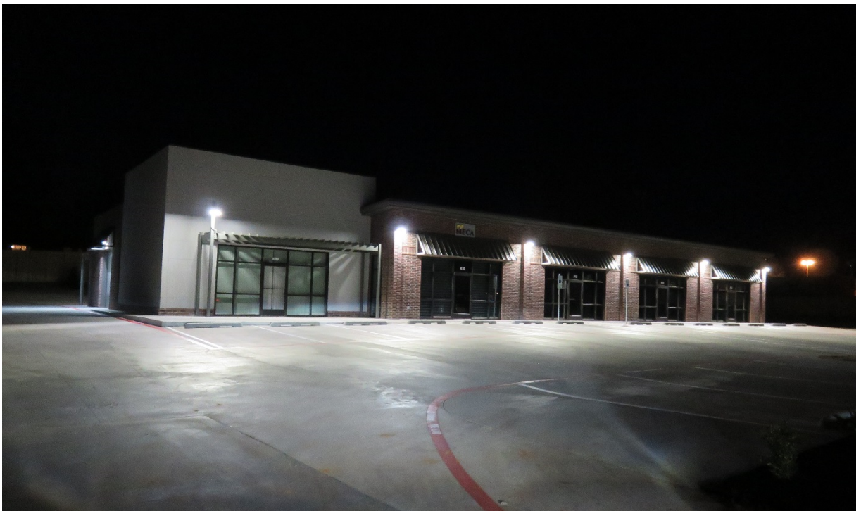
Well Lit parking lot With Security Cameras around Entire Perimeter
