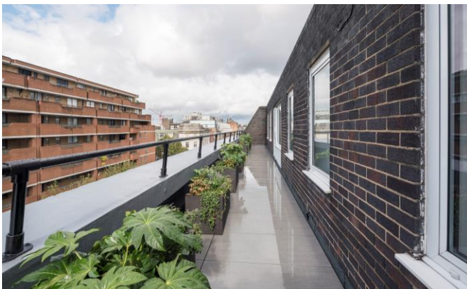
6th floor demised terrace
