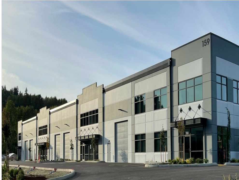
Hoffman Building Exterior
