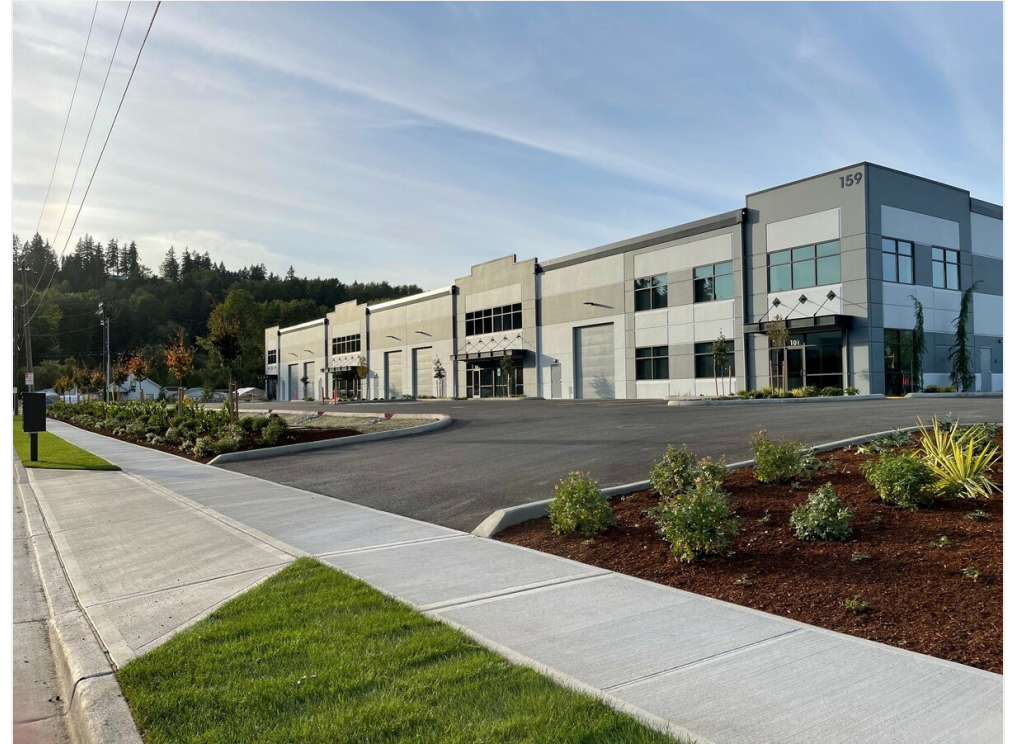
Hoffman Building Exterior
