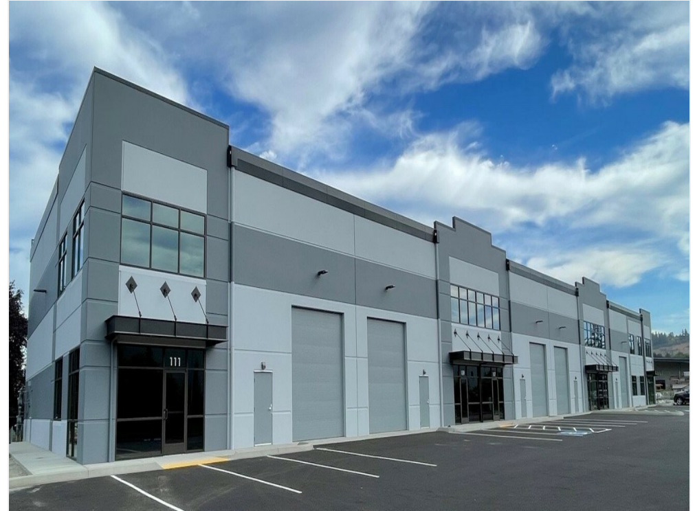
Hoffman Building Exterior
