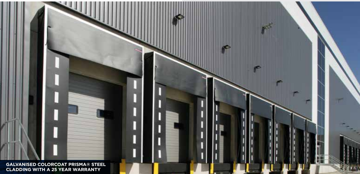
ALL STEELWORK IS PRE-FINISHED WITH A FACTORY APPLIED TWO PART EPOXY COATING
