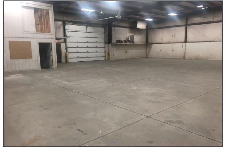
14' Overhead Door in West Bay
