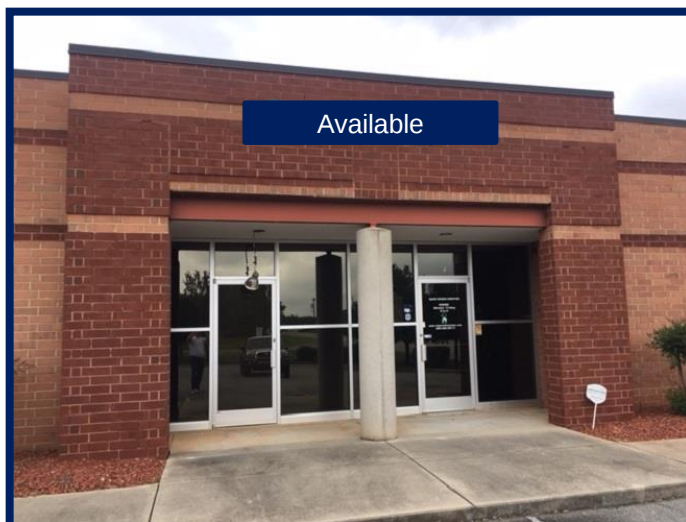
Unit J - 2,392 sf suite This unit has exam rooms with sinks.
