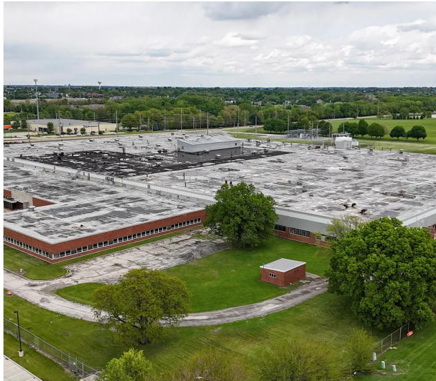
View of north west corner of the property
