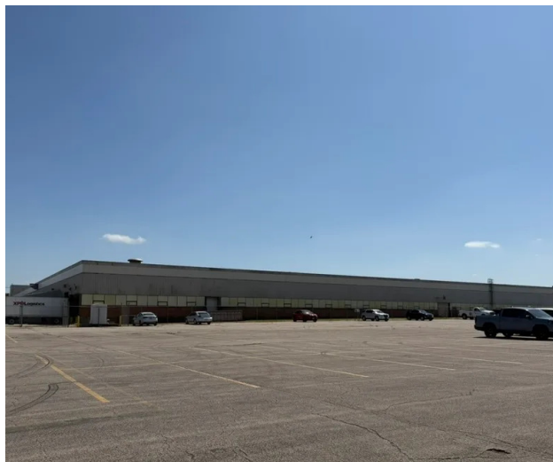
View of the northeast corner from parking lot
