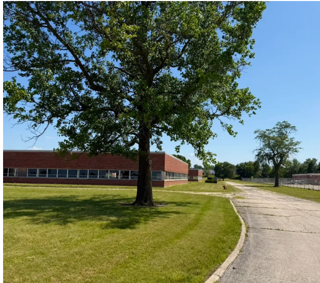
West side of property along Keaton Place
