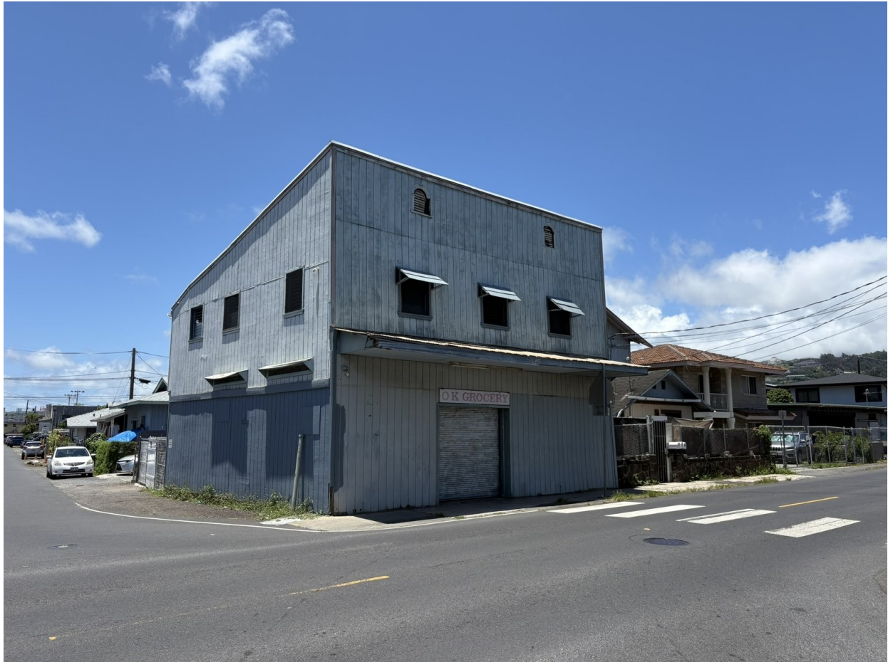
Building A — Corner of Palama Street — Commercial (ground floor) + 4-bed residential (upper)
