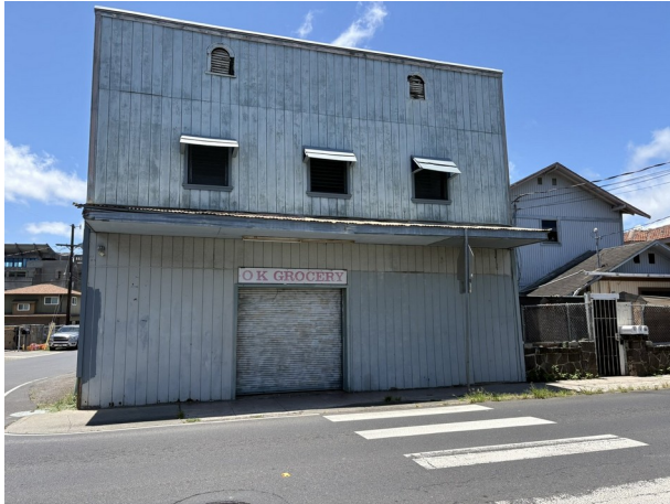
Building A — Front elevation with roll-up door
